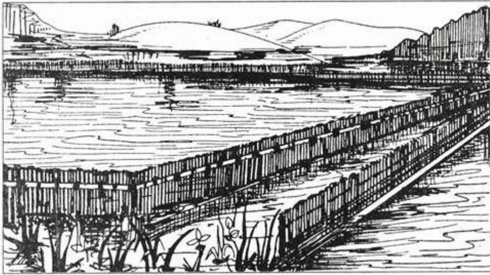
Fig.6 Bamboo Scaffolding enclosers of different size.
